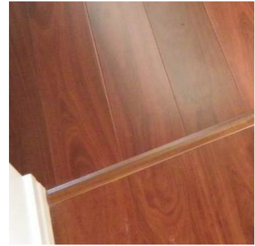
Control joint across a doorway
