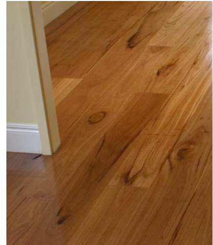
Highly featured High Feature Grade
