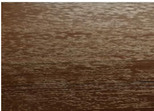
The above photo shows a 2 part water based floor coating after 3 weeks of cleaning with the wrong products.
