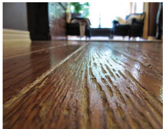
A prefinished timber floor damaged by repeated use of a steam mop cleaner
