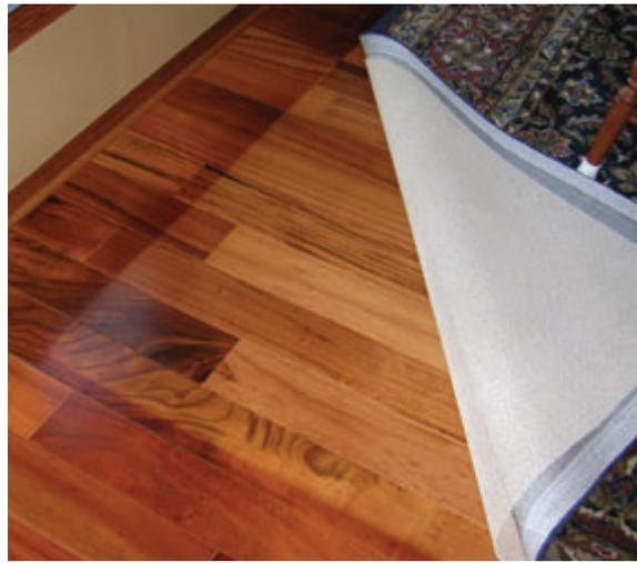
Apply felt to chair legs to protect the floor. Note colour variations where rugs have been covering a timber floor.
