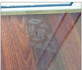
Highly developed prints in the main entrance and note the predominance in one board but also progressing into adjacent boards. Note also the two heal marks facing opposite directions. It appears to have resulted from the person simply walking in and out of the dwelling.
