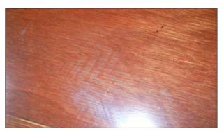
Ghosting does not always appear as foot prints and it does not always appear on horizontal surfaces. In this final example the ghosting appears more predominantly as smudging in the stair risers. In other instances boot prints have been observed in stair risers.
