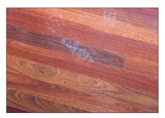
This is the lower storey lounge floor with the photo taken from the upper level. A highly developed boot print as shown in the inset is present in the middle of this floor. Note how areas either side of this area are not affected to a significant degree.
